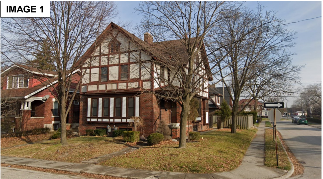
Subject Parcel – 1092-1096 Dougall Avenue – Looking east (Northeast corner Dougall & Pine Street)
